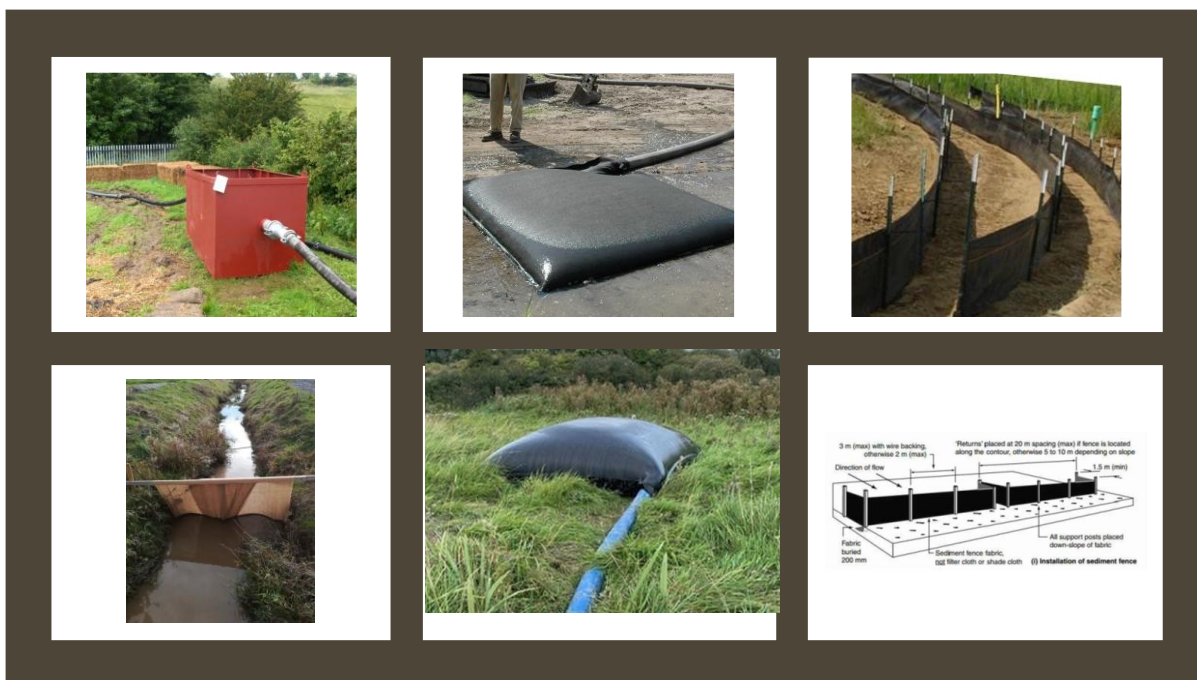
Figure 2-5 Examples of Proprietary Silt Control measures
